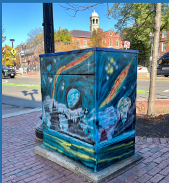
REVITALIZED UTILITY BOXES
